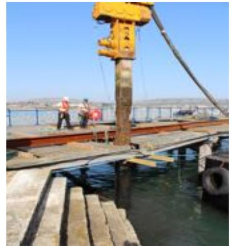
*This photo shows an old pile being extracted - note the middle section showing how it has rotted away. The photo at the top is of a new pile being driven in.*
